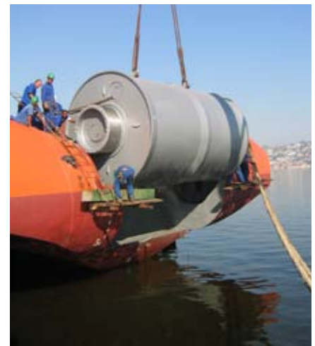
Installing a support roller
