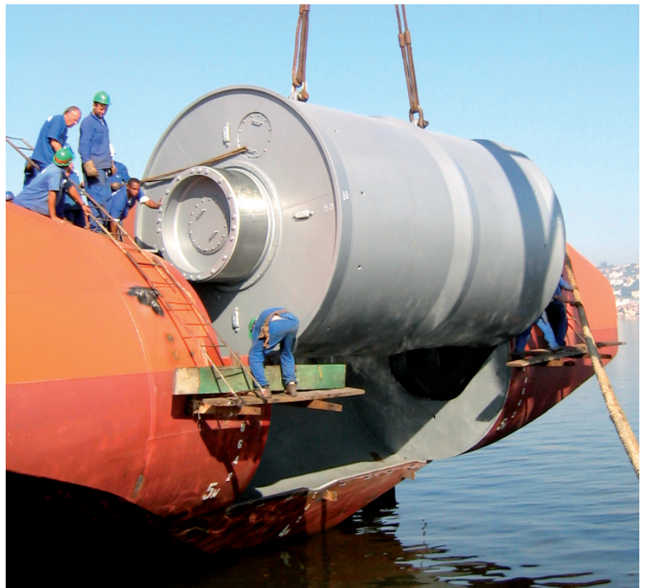
In the present case, the support rollers are not welded by Deform. However, we do take care of the advanced forming.
