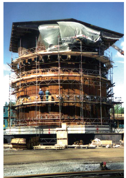
One of many blast furnaces delivered by Deform.
