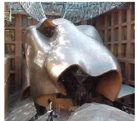
Designed by Frank O. Gehry, the roof of the conference hall in the DG Bank building, Berlin, was formed by Deform
