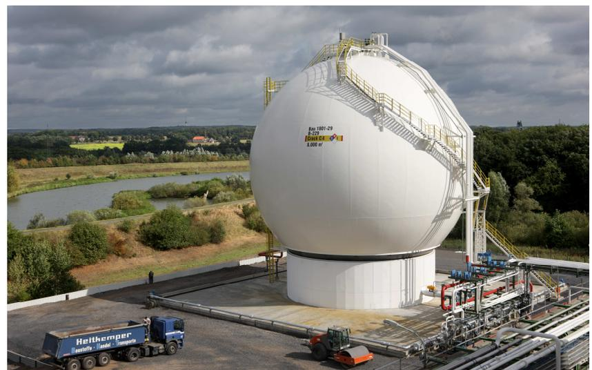
Formed segments welded together to make a complete sphere. Fitting and quality is an absolute requirement. Sphere in the picture is nearly 26 meters in diameter
